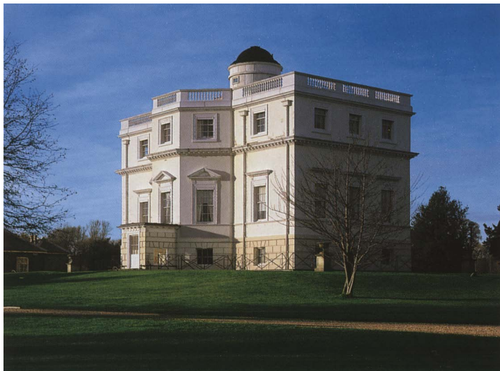
FIG. 13 Richmond Observatory, designed by William Chambers, 1769
