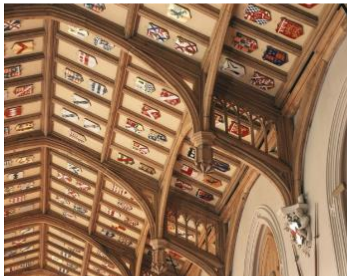
The roof today
