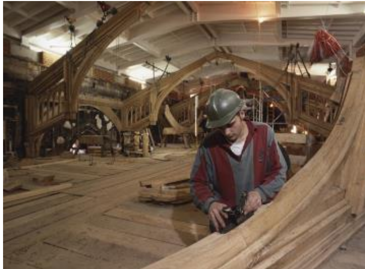
Constructing the hammer beam roof
